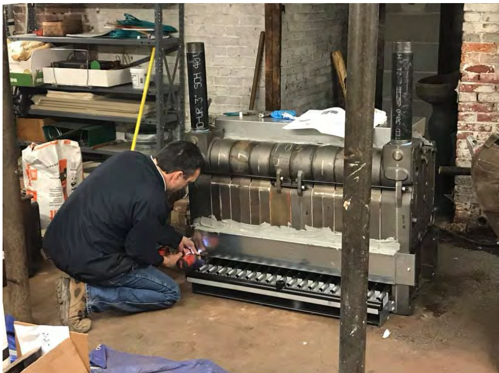
Al Corelli installing new boiler at the Cabot House
